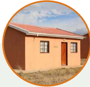
BNG services and top structure
